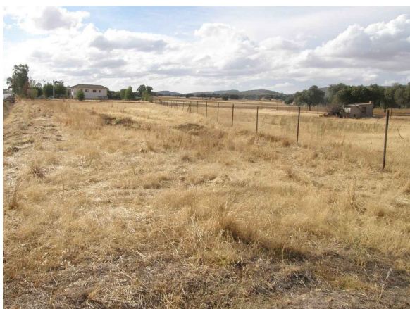
Figure 4.8.2. Road verge with perimeter fence more than 10 m from the roadway in a farmed area. Although rabbits will probably settle here, no impacts on the infrastructure are expected. Photo: Ministry of Development.
