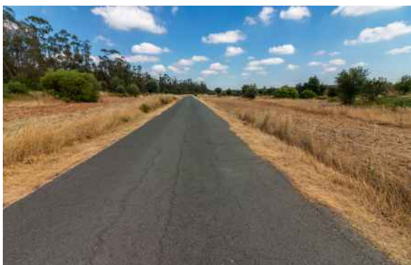
Figure 4.4.1. Verge treatment involving mowing and ploughing to avoid wildfire ignition on a roadside. Photo: Jacinto Román.
