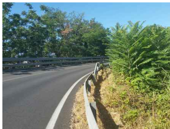
Figure 3.9. Edge of A-8076 road in Coca de la Piñera (Seville), with Ailanthus on the right and Robinia on the left. The colonizing potential of Ailanthus can be appreciated in its fresh shoots (foreground). Photo: Carlos Rodriguez
