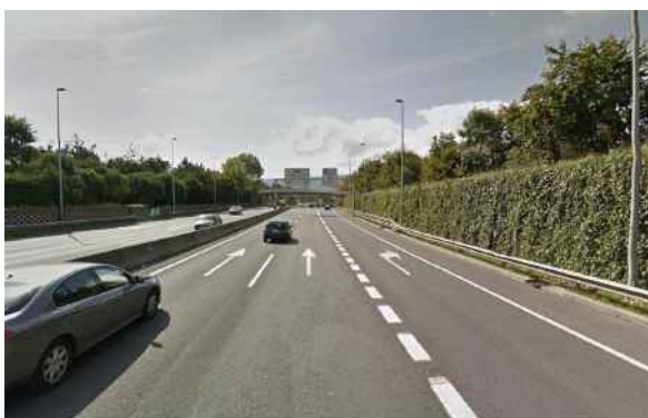
Figure 4.2.1. Highway equipped with infrastructure noise abatement barriers. Subsequent landscaping has improved the aesthetics but has not improved noise reduction. Photo: Basque Government.
