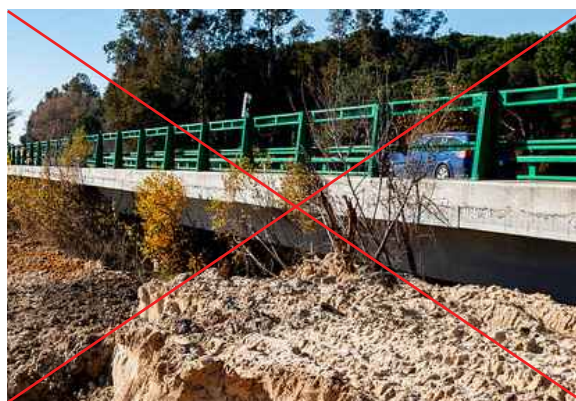
Figure 4.2.2. Conventional bridge replaced by a viaduct to increase the permeability of the infrastructure near Doñana National Park. Unfortunately, the option of sound absorption panels was not contemplated. Photo: Jacinto Román.
