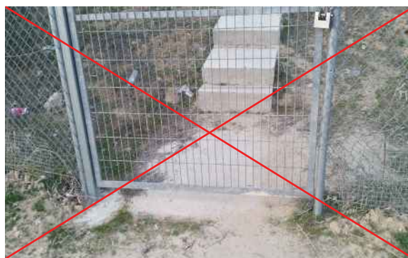
Figure 4.8.3. Example of poorly designed gate in a fence which cancels out the effectiveness of the rest of the measures (buried mesh, double fencing) aimed at keeping rabbits out of a railway embankment. Photo: Carlos Rodríguez.
