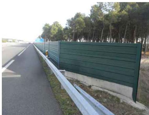
Figure 3.3. Noise abatement panels on the A-601 motorway in Gomezserracin (Segovia). Photo: Government of Castilla y León.
