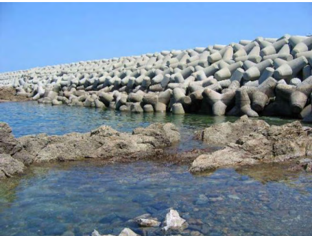
Estructura artificial permeable
