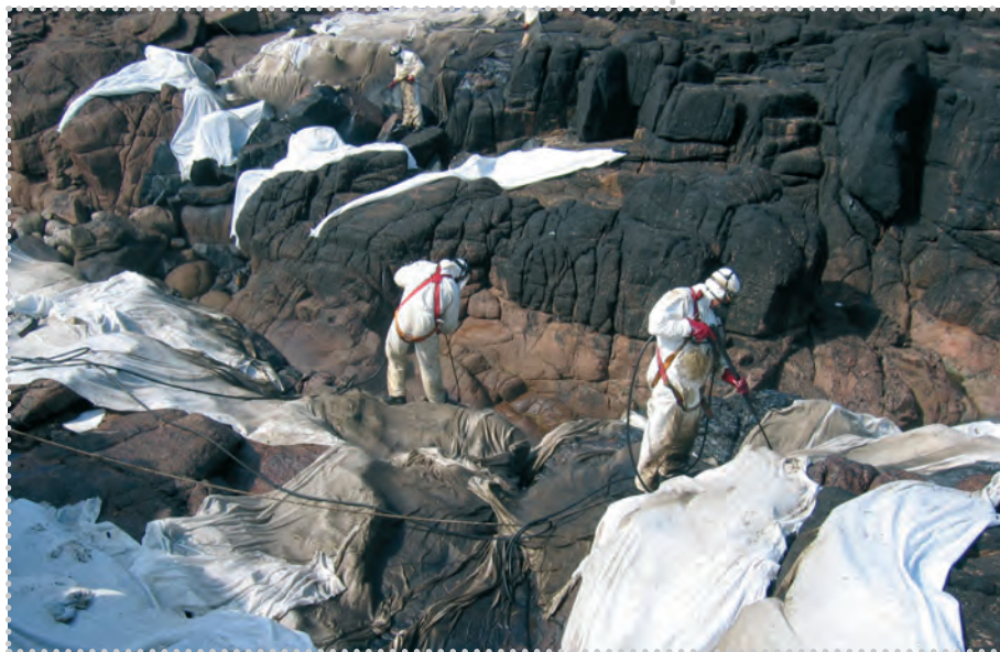
Arrangement of hydrocleaning. Note safety measures and use of absorbent sheets.
