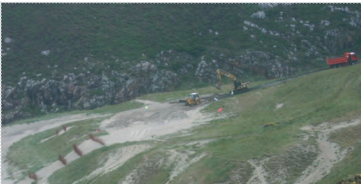
Restoration of dunelands deteriorated by cleanup operations, and removal of a temporary track.
