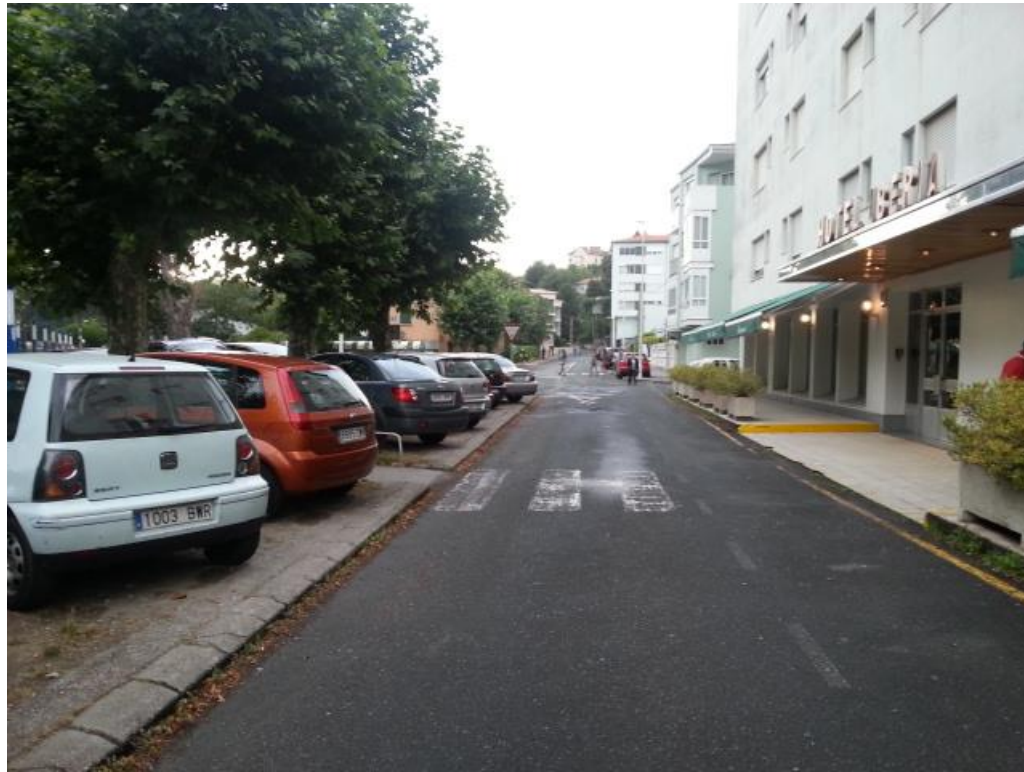
FOTO 5. Tramo colector Cabañas colector C1 PRFV Ø800
