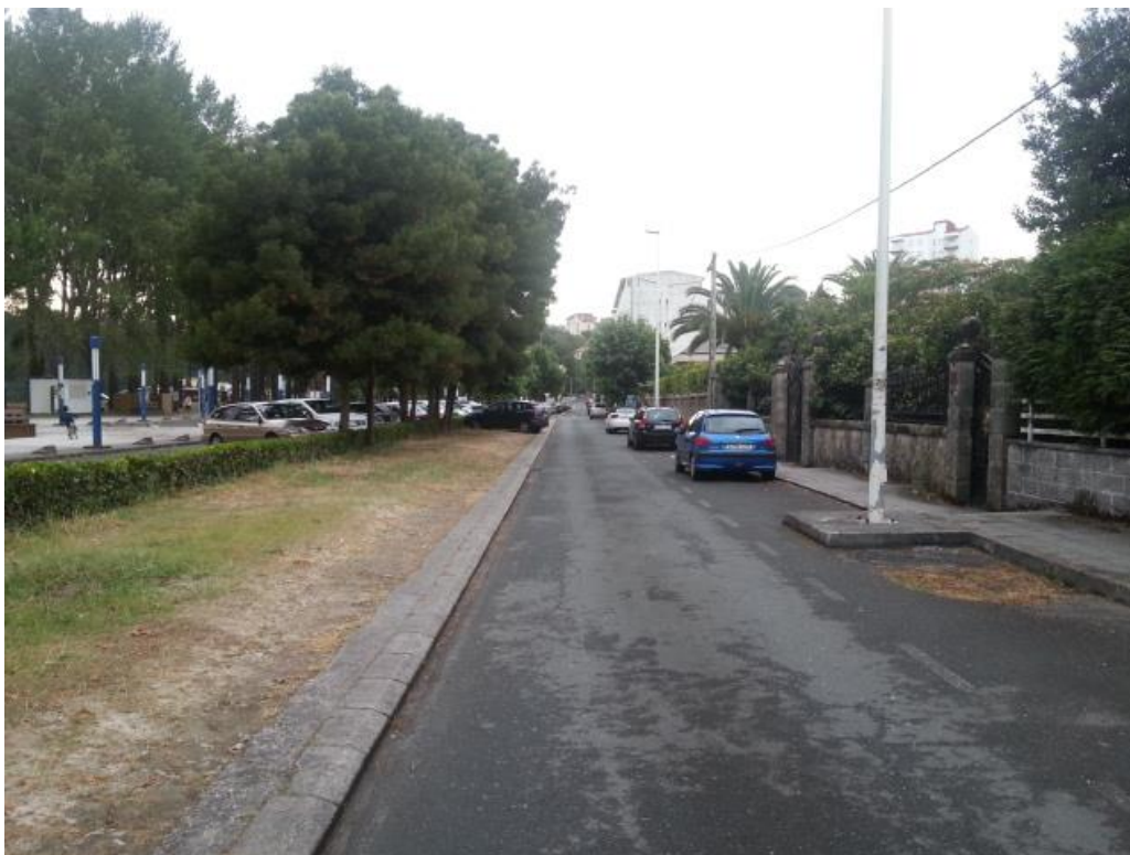
FOTO 6. Tramo colector Cabañas colector C1 PRFV Ø800
